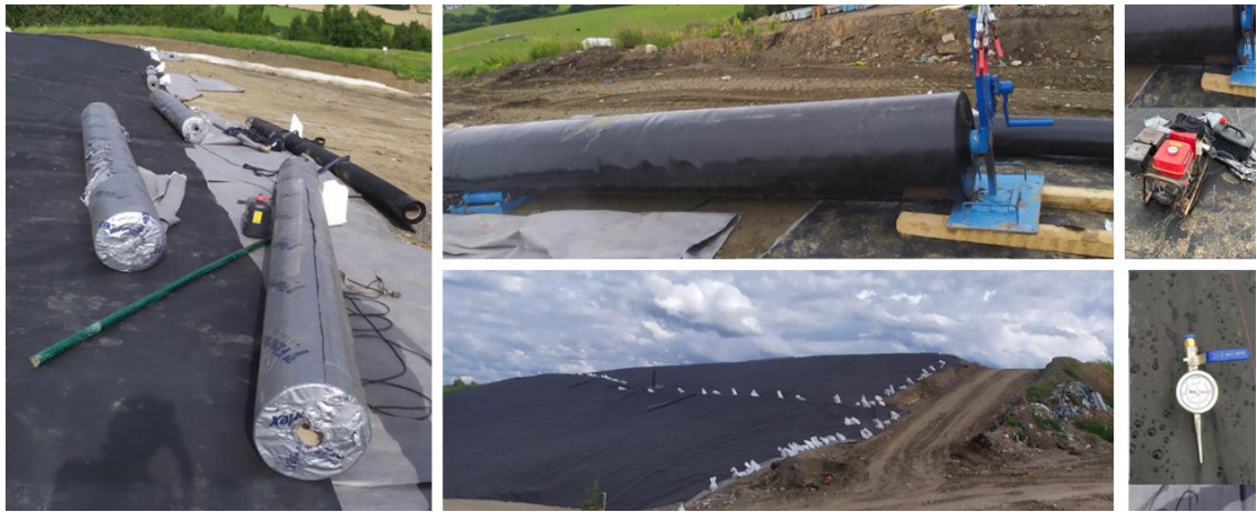
Figure 3.7. Installation of GM during reclamation work (own photos).
